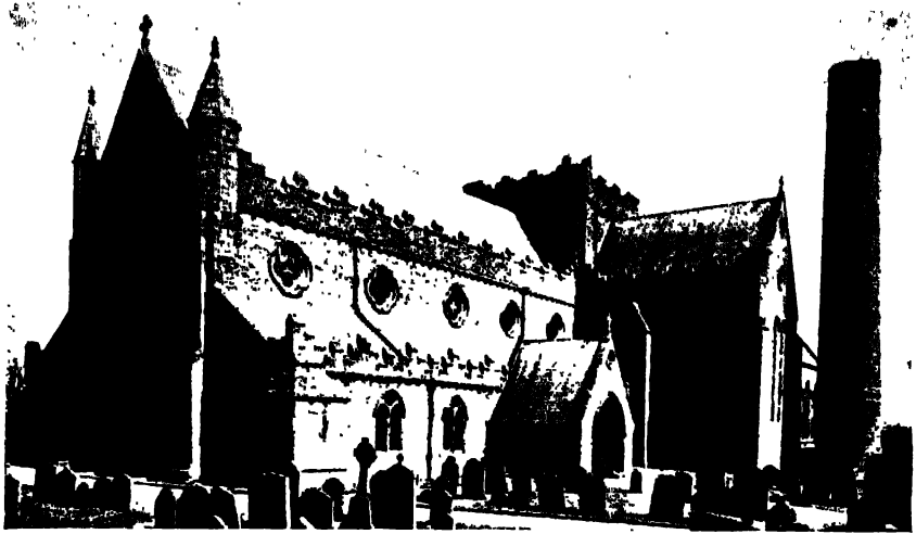
Fig. 170. St Canice's Cathedral, Kilkenny
